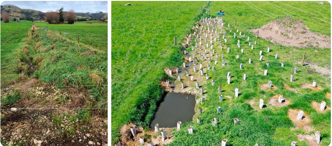
Figure 2. Management approach applied to another farm drain (before left, and after right) – this one has been widened and planted, with a small sediment trap.
